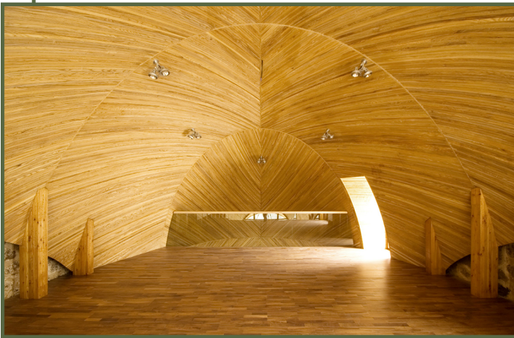
Hardwoods were used throughout the project, with specific materials being selected because of the hyper-saline environment.
